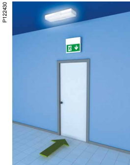
At every exit door planned to be used in an emergency.
